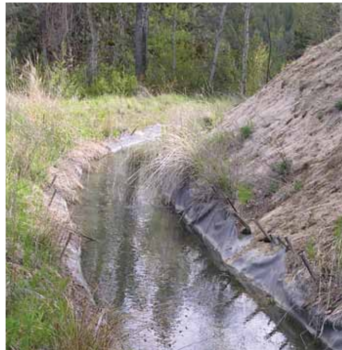
Canal lining and piping can increase irrigation efficiency and free up water that can be sold to conservation buyers for instream use.
