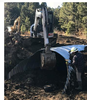
Fish-friendly “stream simulation” culverts like this one allow trout to easily migrate up- and downstream.
