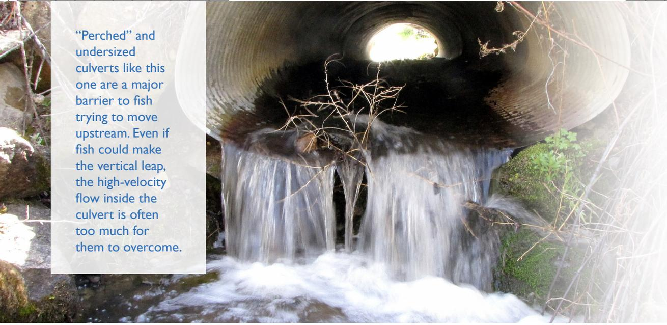
“Perched” and undersized culverts like this one are a major barrier to fish trying to move upstream. Even if fish could make the vertical leap, the high-velocity flow inside the culvert is often too much for them to overcome.
