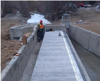
In early December, after weeks of rain, snow, mud, and ice delays, we coordinated installation of a **new corrugated fish screen on Lolo Ditch**. It's a major breakthrough for Lolo Creek, as it prevents the loss of more than *10,000 fish each year* in the ditch, and ends a 17-year wait on this high-priority project. We're hopeful, too, that the screen will help boost trout numbers in the currently fish-depleted lower Bitterroot River.
