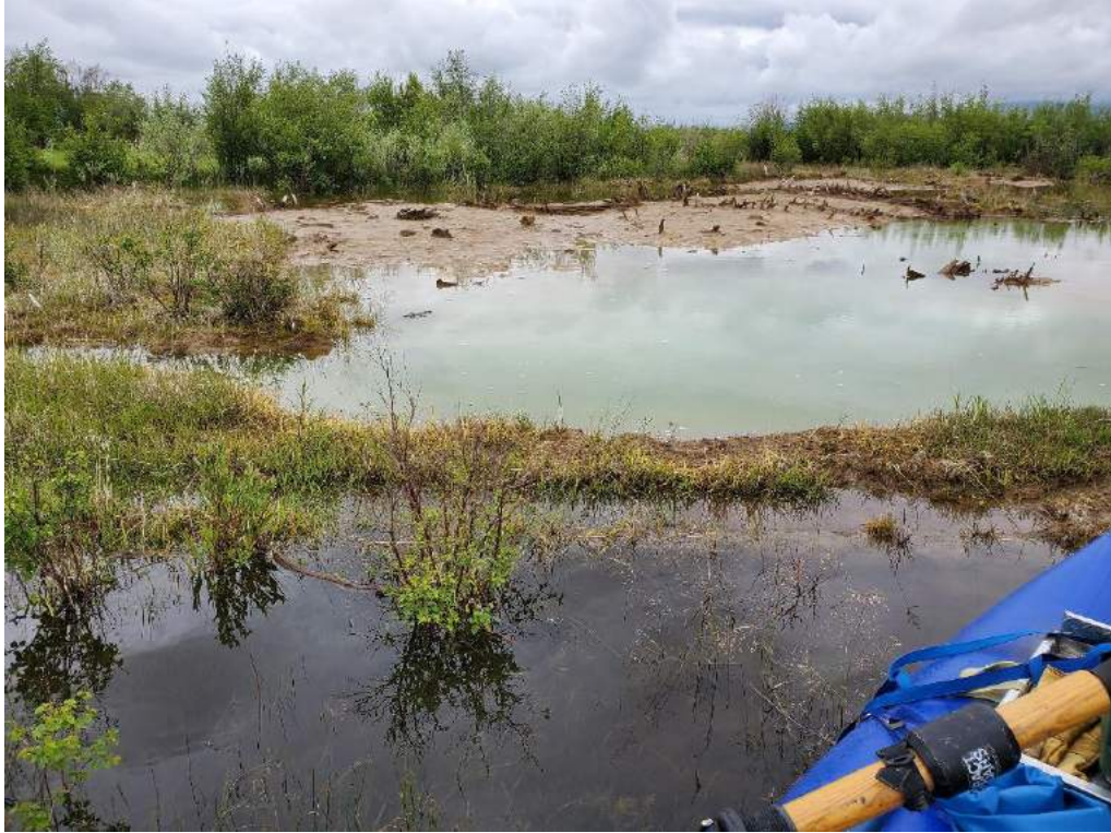
Figure 5. Partially-functioning berm on slicken #4. The berm contains some contaminated water, but is in danger of being overtopped during high river flows.
