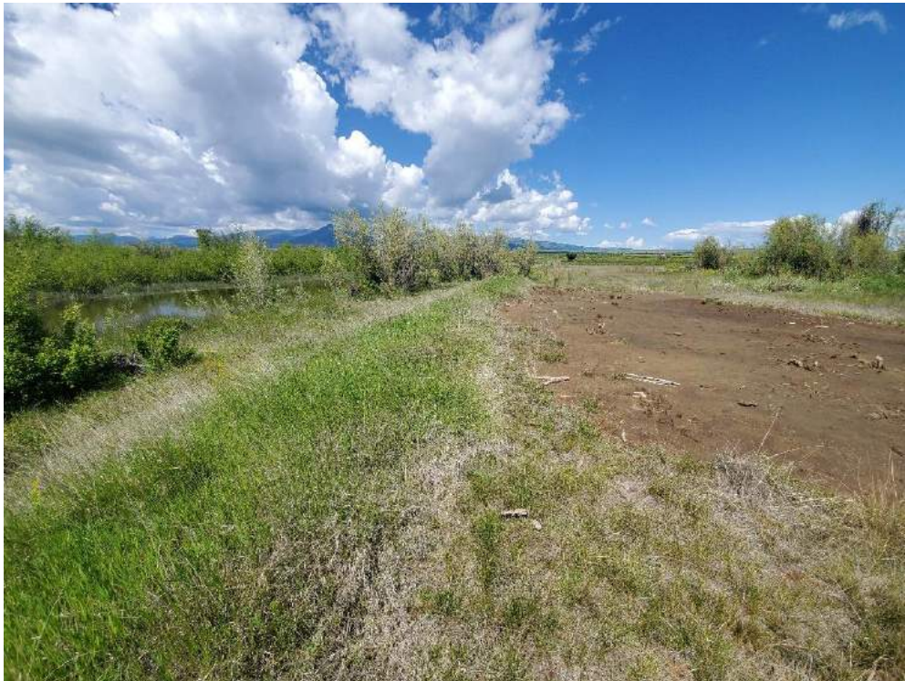
Figure 7. An intact berm on slicken #94. Note that the berm is vegetated and keeps slicken material out of the river (on the left).
