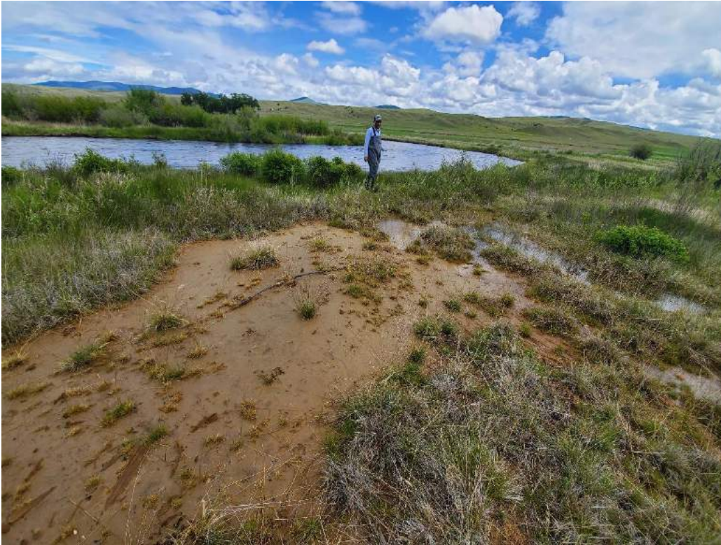
ID#31, SER=2, AR=2: A good example of a berm keeping contamination from contacting the river.
