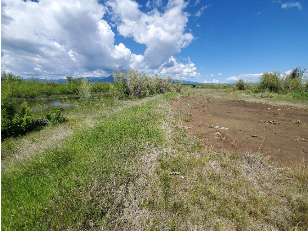
Figure 7. An intact berm on slicken #94 in Phase 12. Note that the berm is vegetated and keeps slicken material out of the river (on the left).
