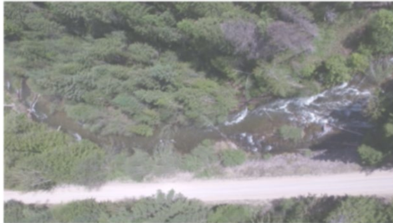
Cedar Creek Road limits floodplain connection—2018
